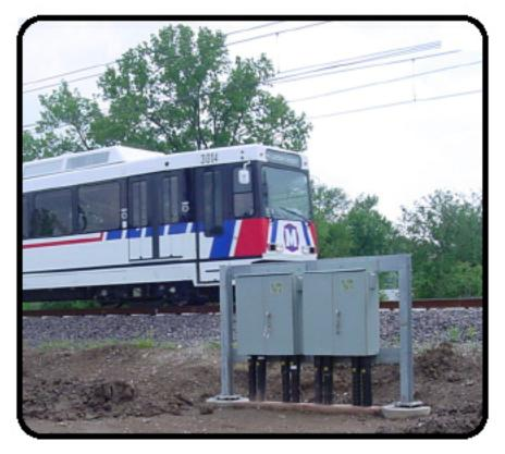
TYPICAL POWERSWITCH FIBERGLASS ENCLOSED DISCONNECT SWITCHES CONNECTING CABLES TO OVERHEAD CONTACT SYSTEM SUPPLYING TRACTION POWER TO THIS MODERN TRAIN. EACH ENCLOSURE HOUSES TWO 2000 AMP, 1000 VDC FEEDER SWITCHES AND ONE 2000 AMP TIE SWITCH.
